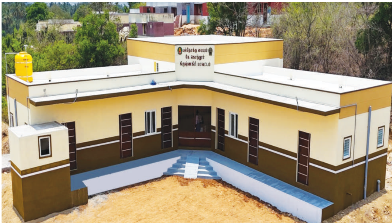
Tribal Multipurpose Centre, Krishnagiri District.
